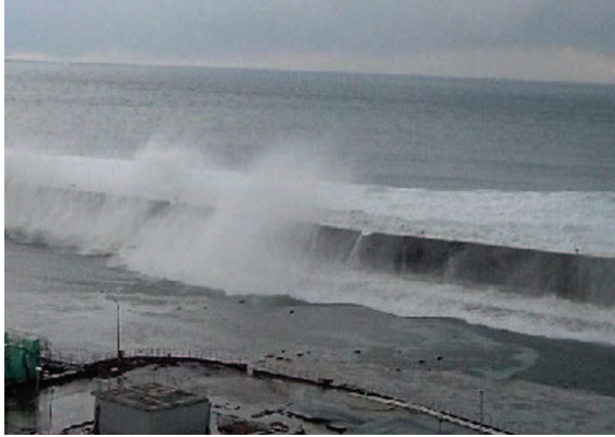
Figure 12: Sea wall breach.
